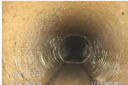
Mainline Camera View
